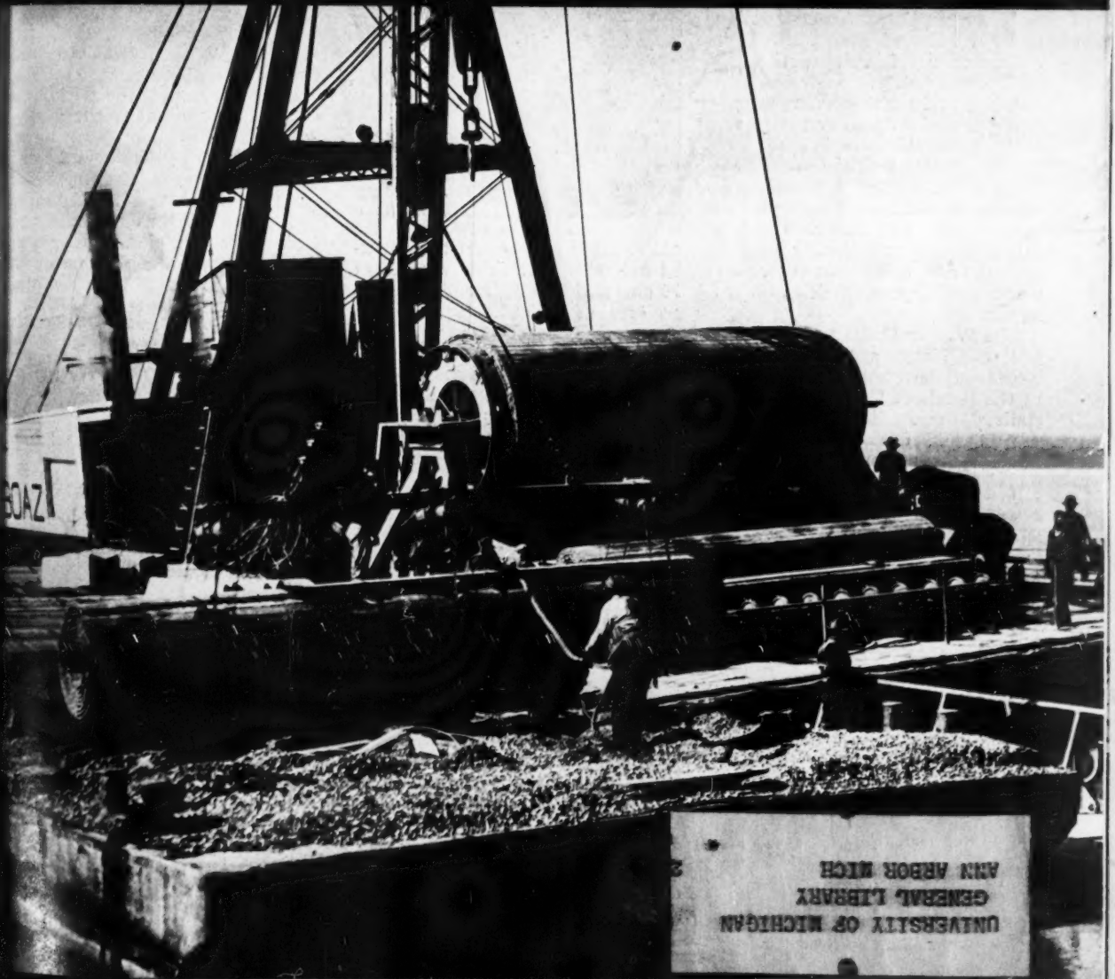
New type of flexible reinforced-concrete mattress for Mississippi River revetment.
